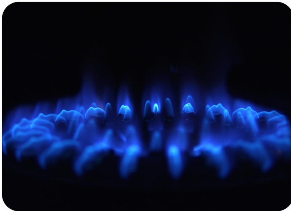
The blue flame in this photo is burning inside a home furnace. The fuel is natural gas, and it combines with oxygen when it burns. This chemical reaction, called a combustion reaction, gives off a lot of energy.
